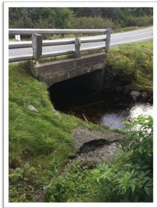
Figure 2: Concrete Culvert - Marine Drive
