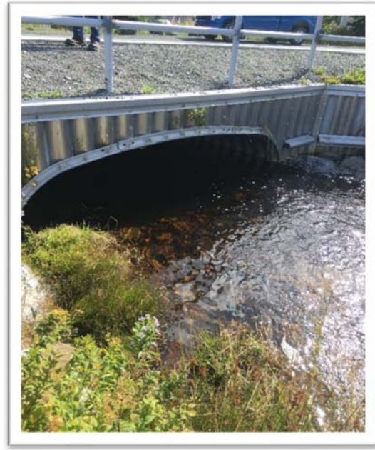
Figure 1: Arch Bottomless Culvert - Lynch's Lane
