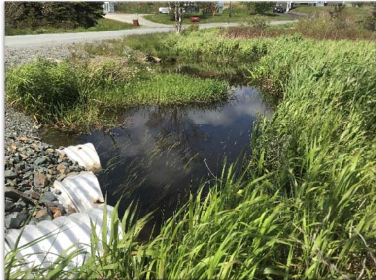
Figure 25: Triple 600mm CSP Culverts on Crowe's Lane
