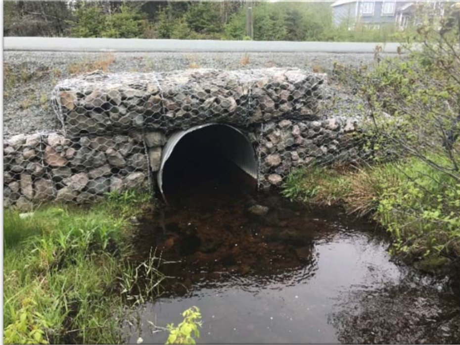
Figure 5: Existing 1200 CSP Culvert Western Island Pond Drive
