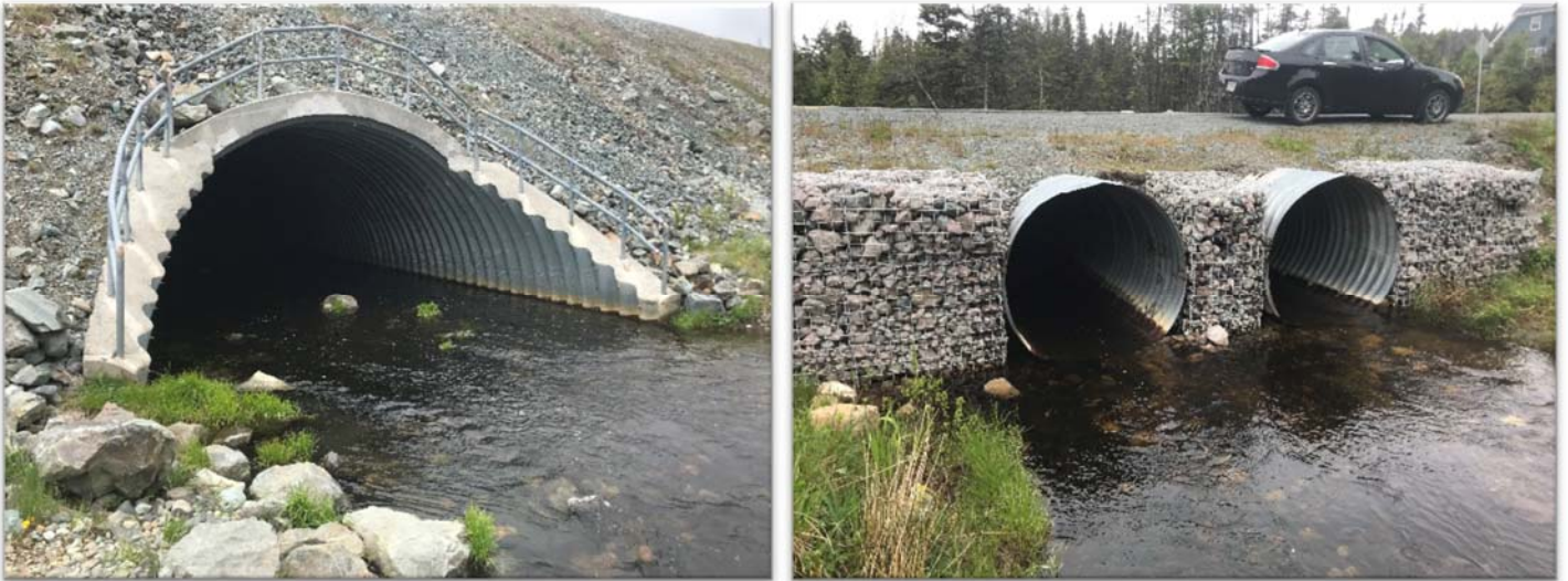
Figure 16: Culvert Structures on Torbay Bypass Road and Rattling Brook Road
