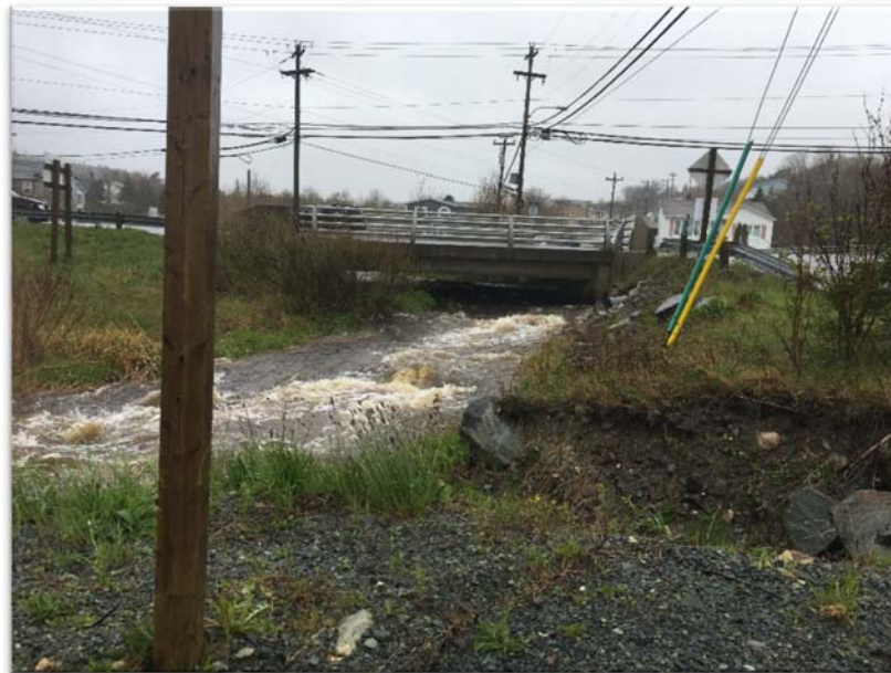
Figure 17: Bridge Structure - Torbay Road during May 30, 2018 Storm Event
