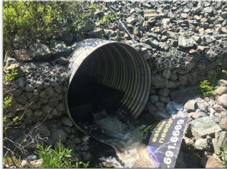
Figure 28: 2000mm CSP Culvert - Torbay Road
