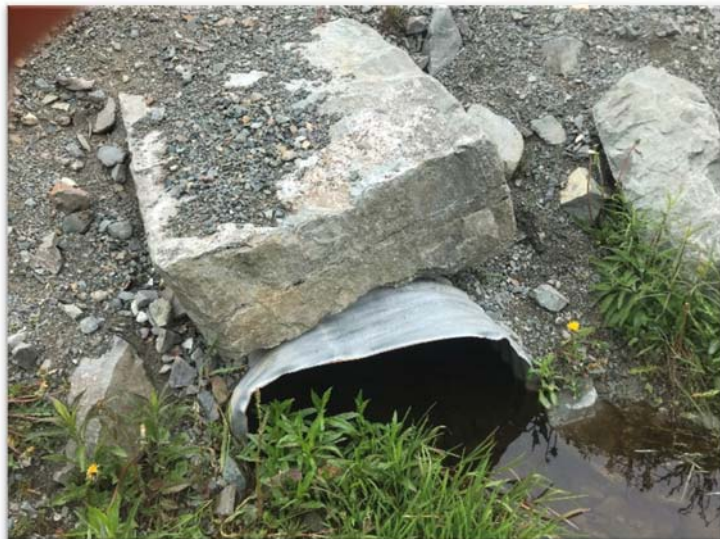
Figure 29: Rock Compressing Culvert - Rosebud Street
