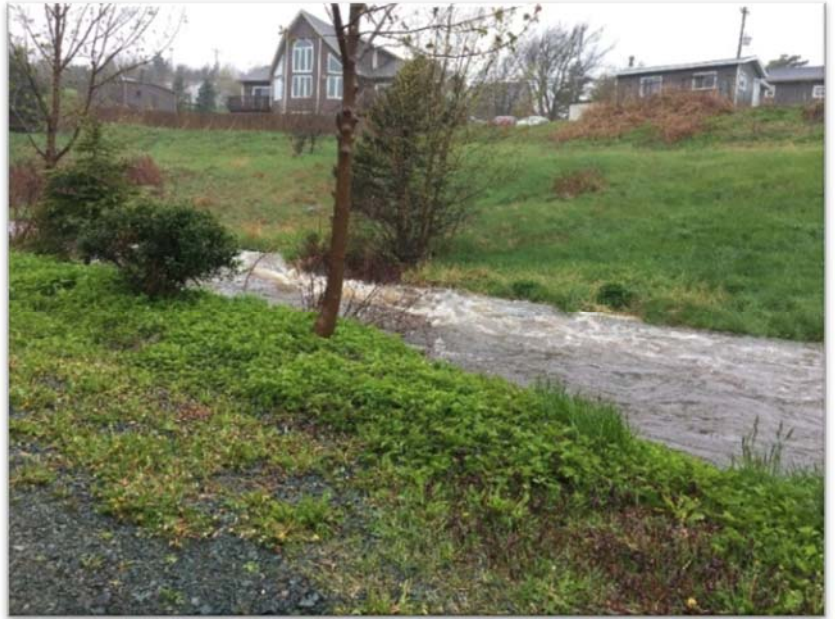
Figure 14: Stream Approaching Capacity During Heavy Rainfall Event
