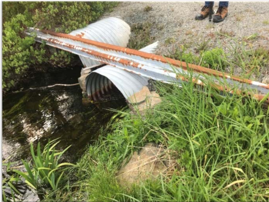
Figure 15: Twin 900mm CSP Culverts – Woodfine’s Lane
