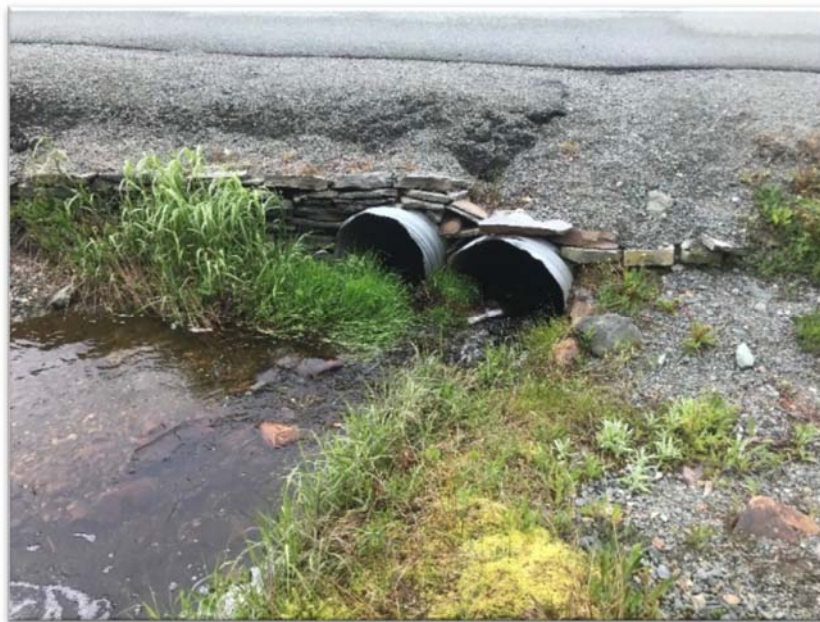
Figure 4: 600 & 700mm CSP Culverts - Skipper's Landing
