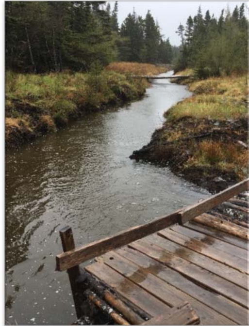
Figure 3: Skipper's Landing Cutoff Drainage Ditch
