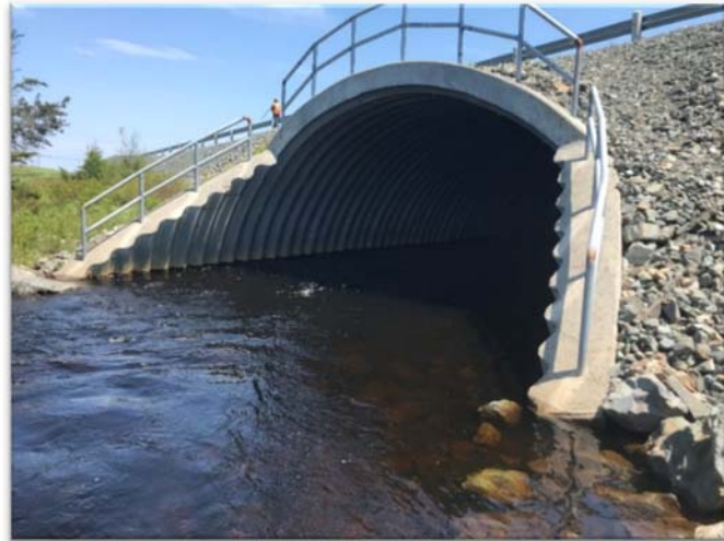
Figure 11: Large Culvert Structure - Torbay Bypass Road
